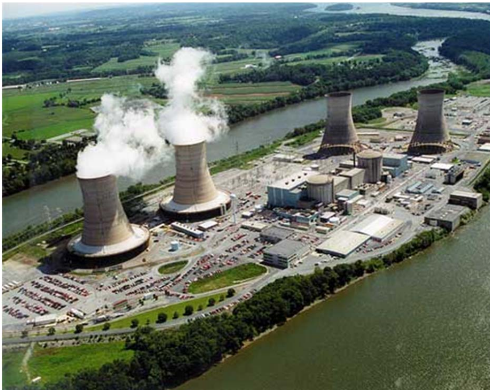
Three Mile Island, on the Susquehanna River at Harrisburg, Pennsylvania. On the right is mothballed Unit 2, which almost completely melted down in 1979, and is now owned by FirstEnergy. Unit 1, to the left, is owned and operated by a subsidiary of Exelon Corp.
